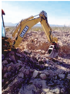
Digging the trench for storage pipe
