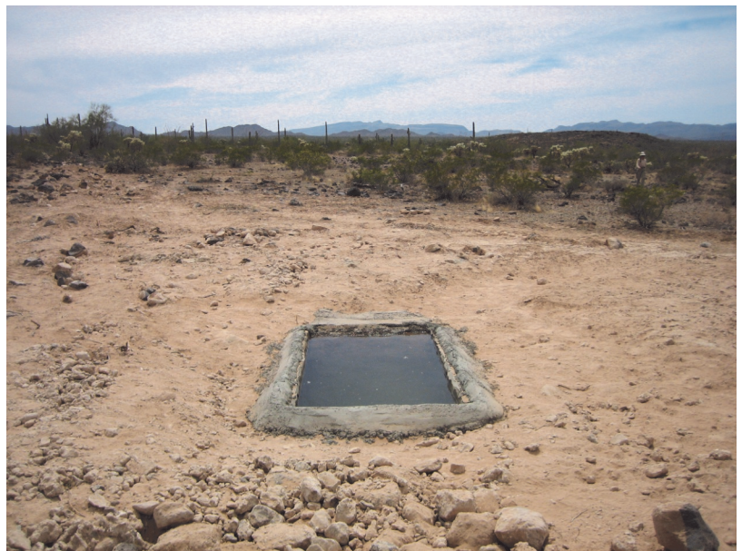
Finished trough full of water
