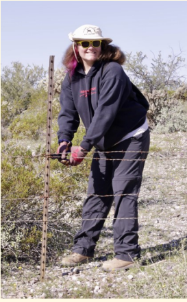
L-Following behind Al, Bo removes clips from a t-post so the barbed wire can be lowered to the ground.
